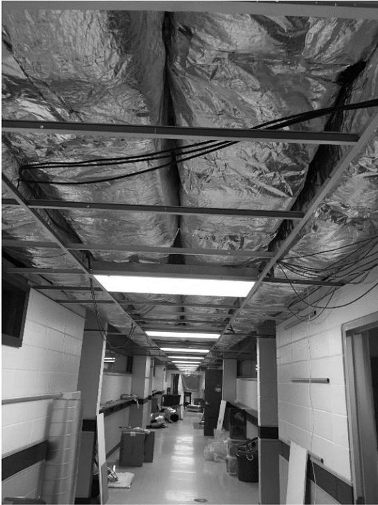
The hallways are cluttered with construction debris. The ceiling tiles have not yet covered up the long runs of insulated ducts.
