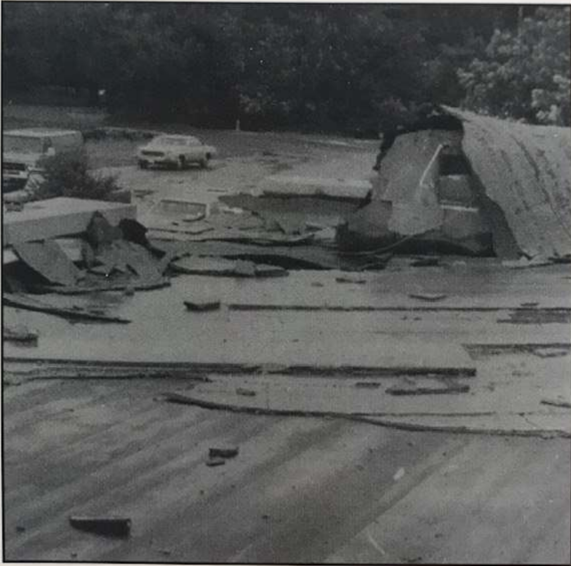
Tornado damage to school
